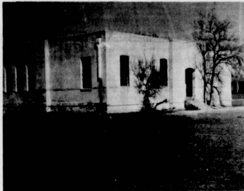
INADEQUATE FACILITIES -- The old West Ward cafeteria, left, and the field house at Tiger Stadium are examples of inadequate building facilities for Slaton schools. The field house is used only by visiting teams, and dressing room and restroom
