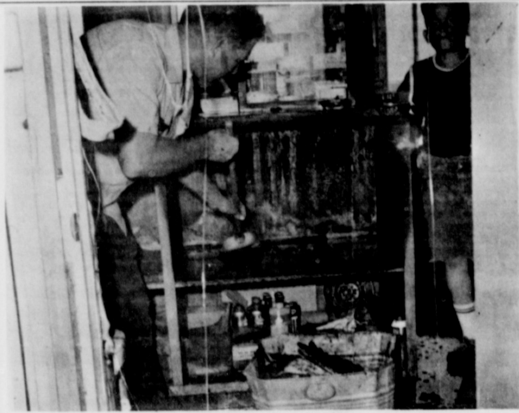
FIRE CAUSES SLIGHT DAMAGE — A Tuesday noon fire at The Dutchman, located west of town on the Union Road, resulted in minor damage to a counter, some smoke damage to two shelf walls and melted a neon sign. Hugo Mosser, owner, shown cleaning out debris, said the fire started in a waste basket. The alarm was answered by two units of the Slaton Volunteer Fire Department, but the blaze was under control before firemen arrived. (SLATONITE PHOTO)
