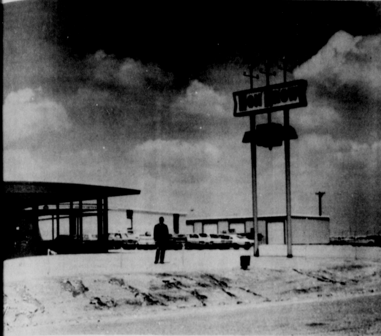
VIEW OF NEW CHEVY CENTER, BODY SHOP IN BACKGROUND
