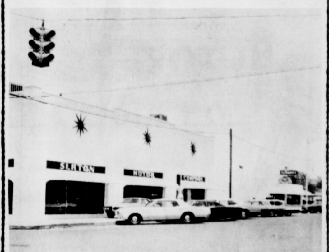
NEW AUTO CENTER--Slaton Motors, Inc., new Oldsmobile-Pontiac agency in Slaton, is holding a formal opening Friday and Saturday at 130-150 W. Lynn. The center brings together Davis Olds, Bownds Body Shop, and Kendrick Pontiac under a new agency. All citizens are invited to the formal opening.
