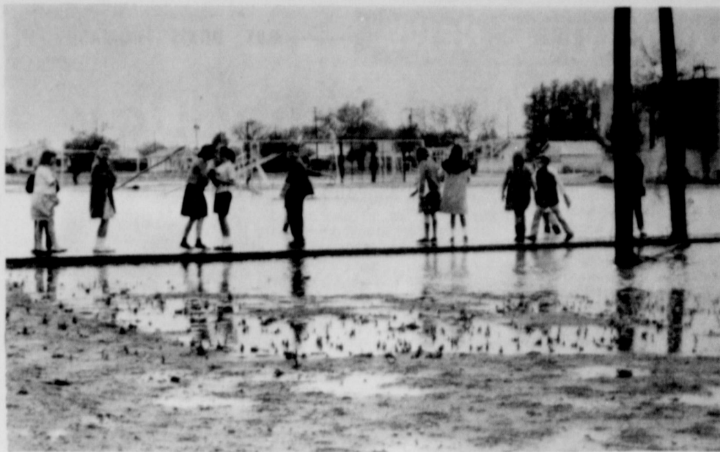
SIDEWALK HELPS — It was hard for West Ward students to keep their feet dry Monday afternoon after school, but the newly-constructed sidewalk leading out the back door of the school
