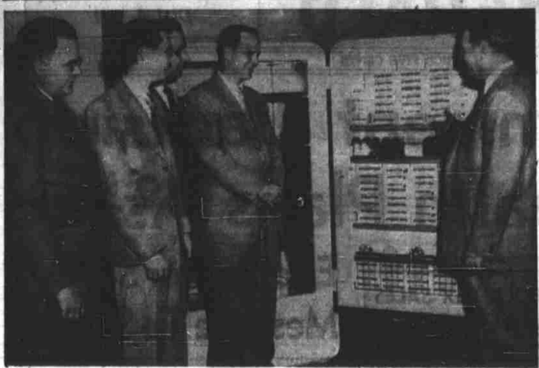
Inspect New Lines
