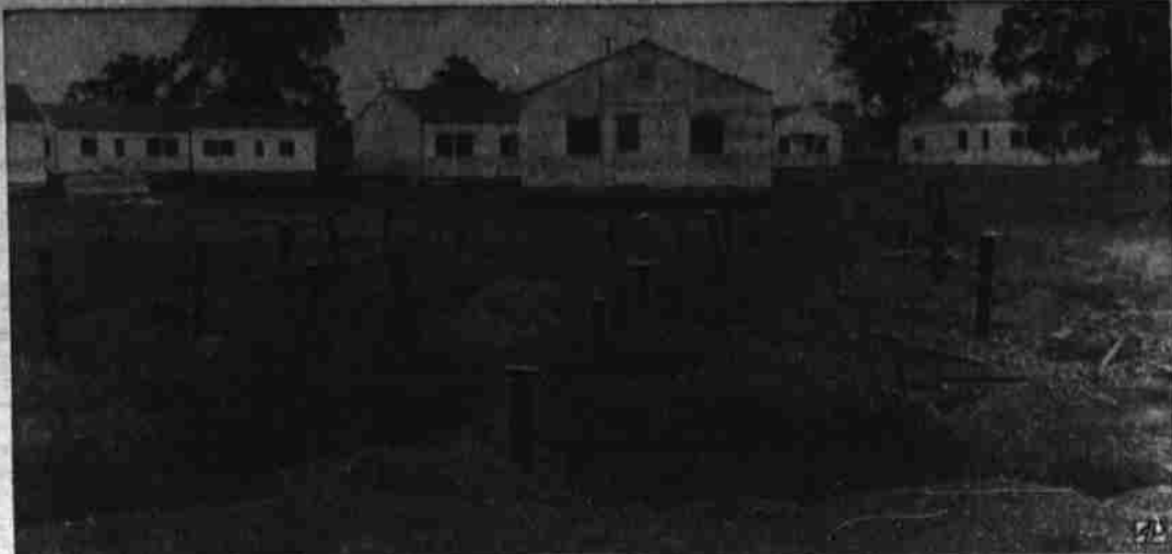
HOMES SPEED-UP —Prefabricated houses, part of a 650-structure project at Indianhead, Md., will soon cover these plings. The houses can be quickly assembled and dismantled.
