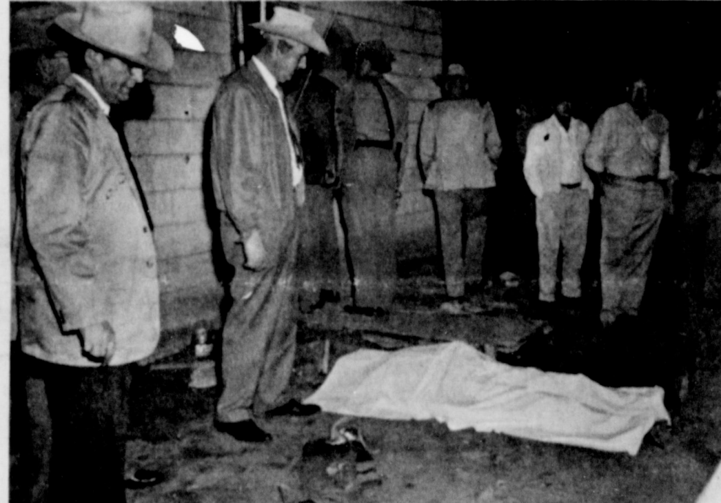
SCENE OF GUN BATTLE--Shown above is the concrete building in which Chester Tatum, 55, barricaded himself against officers in an hour-long gun battle Monday afternoon. The body of Tatum lies on the ground after he was removed from the house, fatally wounded in the chest. At left is Garza County Sheriff L. E. Clayborn and immediately to his right is Garza County Deputy Elton Corley. Other patrolmen and onlookers are unidentified.
