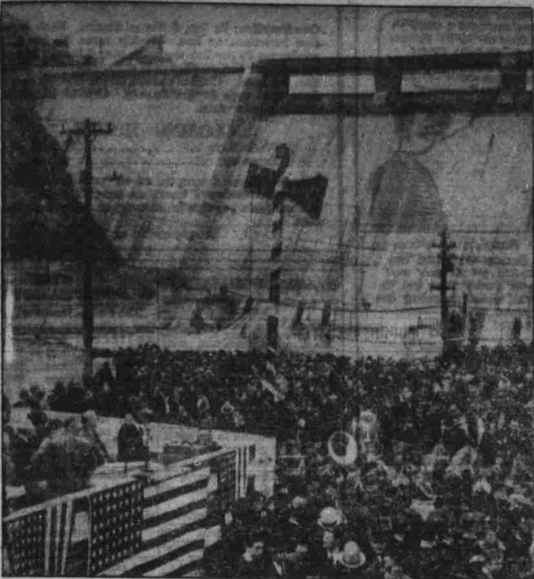
While thousands of persons watched and cheered sluice gates of Norris dam in Tennessee, the world's fourth largest, were closed in a ceremony marking formal completion of the prize project of the TVA. President Roosevelt, from Washington, pressed a key which set off a siren, signal to the celebrators at the dam, some of whom are shown above. (Associated Press Photo)
