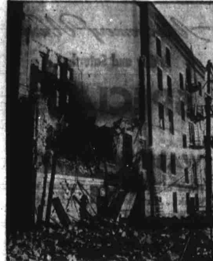
LANDMARK REDUCED TO SHELL—Only the walls are left of the Truop Hotel, five-story landmark burned out in Topeka, Kas., by fire that spread quickly and routed occupants, all of whom police said apparently escaped unhurt.
