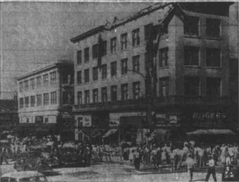
Bakersfield Quake Damage
