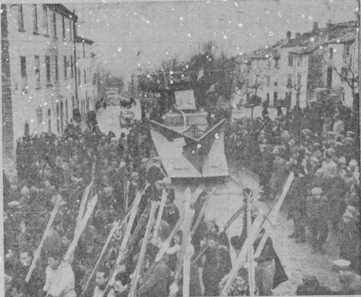
VILLAGERS WELCOME THEIR GIFT—Turning out for the arrival of an American snow plow, the residents of the tiny mountain settlement of Capracotta, Italy, give it a big welcome. The plow is a gift from the residents of Jersey City, N.J., and skiers from the town are leading the way toward a road in the Apennine Mountains where it was given a try-out.
