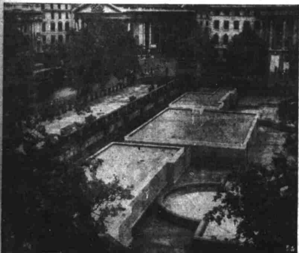
NO TOURIST SPOT NOW —Travelers who've "done" London might have trouble recognizing Trafalgar Square as it is now, with these public brick and concrete air raid shelters squeezed into the square. At the upper left background is St. Martin's in the Field church. The National gallery is located to the left, the Nelson monument to the right.
