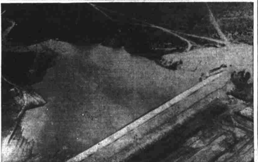
WATER FOR THE CITY is shown impounded in the Powell Creek lake (above) and the Moss Creek lake (below) after brisk thundershowers in this area Sunday night. The Powell lake level is just four feet above the scarp spillway at extreme left. Depth of the water is 21 feet at the dam. The Moss Creek lake, which caught its first water, has 11 feet and can take 24 feet more. The views were snapped from a plane piloted by Art Wintheler, municipal airport manager. (Kelsey Photos).
