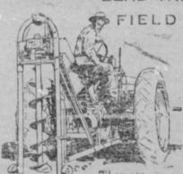
attach on any farm tractor with rear end power cake-off. Digs holes in hard dry soil It's easy to set the depth gauge and control all operations from the driver's seat. Interchangeable auger sizes . . . Timken bearings.
