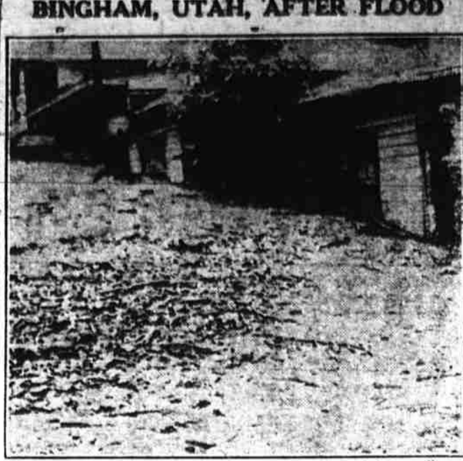
Many houses in Bingham, Utah, were buried almost to their eaves by rocks and mud when a heavy rain at the head of Bingham canyon sent a flood down the narrow gulch in which the town is located. Four years ago a snowslide took 37 lives in the town.
