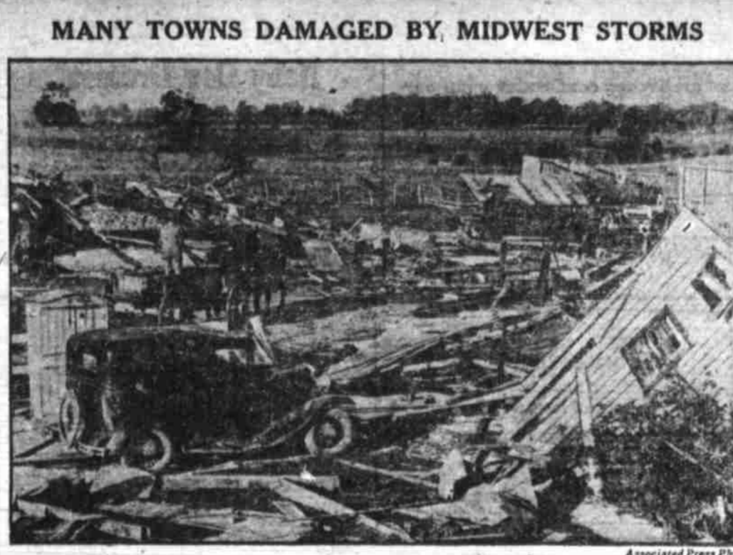
Tornado-like winds have caused widespread property damage in several towns of midwestern states. Typical of such wreckage was this scene at Vernon, Ind., where several were injured by a storm.
