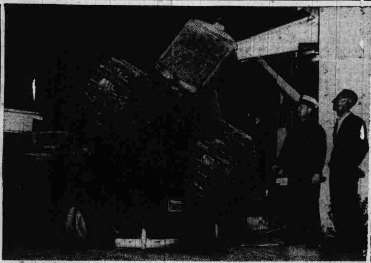
RUNAWAY BULLDOZER HITS CAR—A runaway bulldozer belonging to the City of Dallas lumbered driverless for four blocks, veered through a fence, ripped off the corner of E. P. Simms' house, climbed on top of his auto and stalled (above). Police Sergeant D. J. Cameron said that youths playing with the machine where it was parked in a vacant lot started it on its trip. (AP Photo.)
