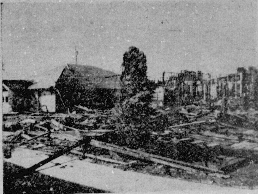
Pictured above is all that remained of the East Cisco Baptist Church after the devastating fire last week. Officers announced that a drive for funds to rebuild the structure would begin at services Sunday.
