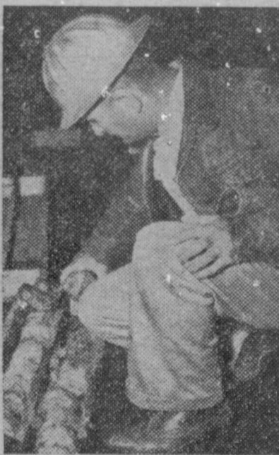
ON FLOOR OF RIG at right, Lone Star geologist saves "core" of well being drilled. "Core" reveals information vital to proper completion and operation of well.
