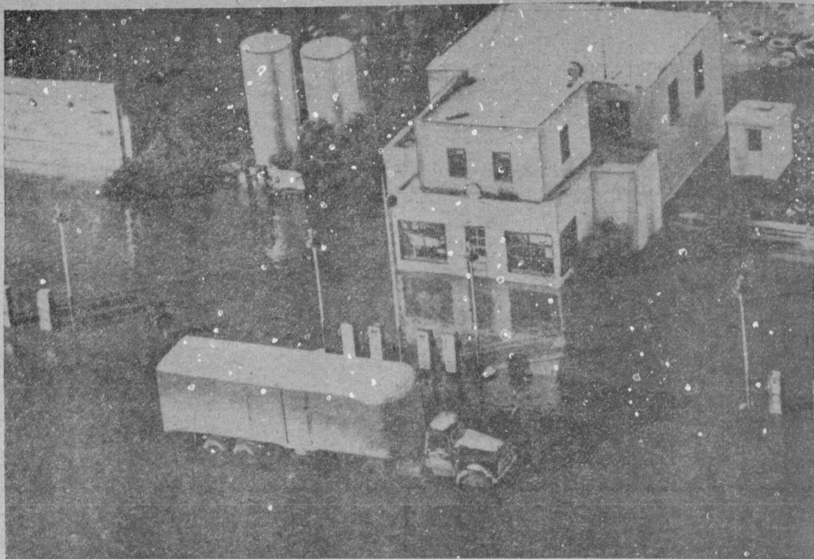
FULL FILLING STATION —This filling station on U.S. Highway 66, near Valley Park, Mo., would be happy to trade its gasoline pumps for one that works with water. The transport truck was abandoned by the driver when it stalled in two feet of water from the overflowing Meramec River. Flooded river basins in Illinois, Indiana and Missouri left nearly 4000 persons homeless.
