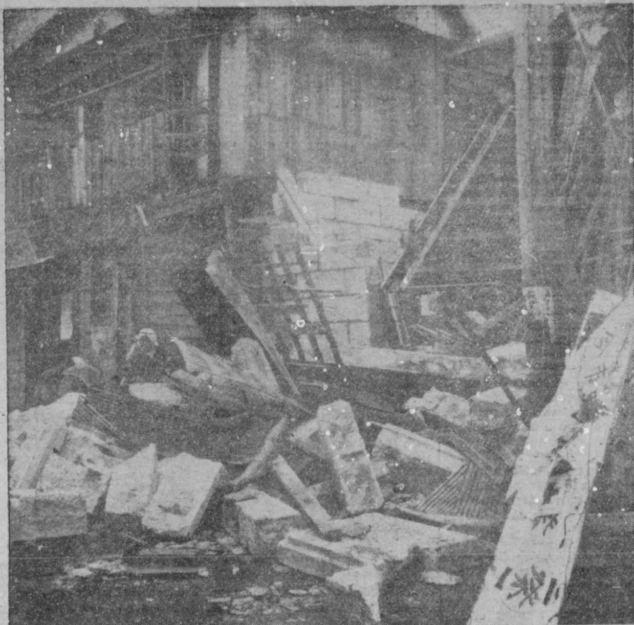
HARD HIT --The worst earthquake Japan has experienced since the Tokyo disaster of 1923 has now destroyed 874 houses. More than 5000 other houses were partially damaged by the wave of three quakes. Hardest hit was the town of Imaichi where 80 per cent of the dwellings suffered damage, and stone houses like the one shown here were demolished.
