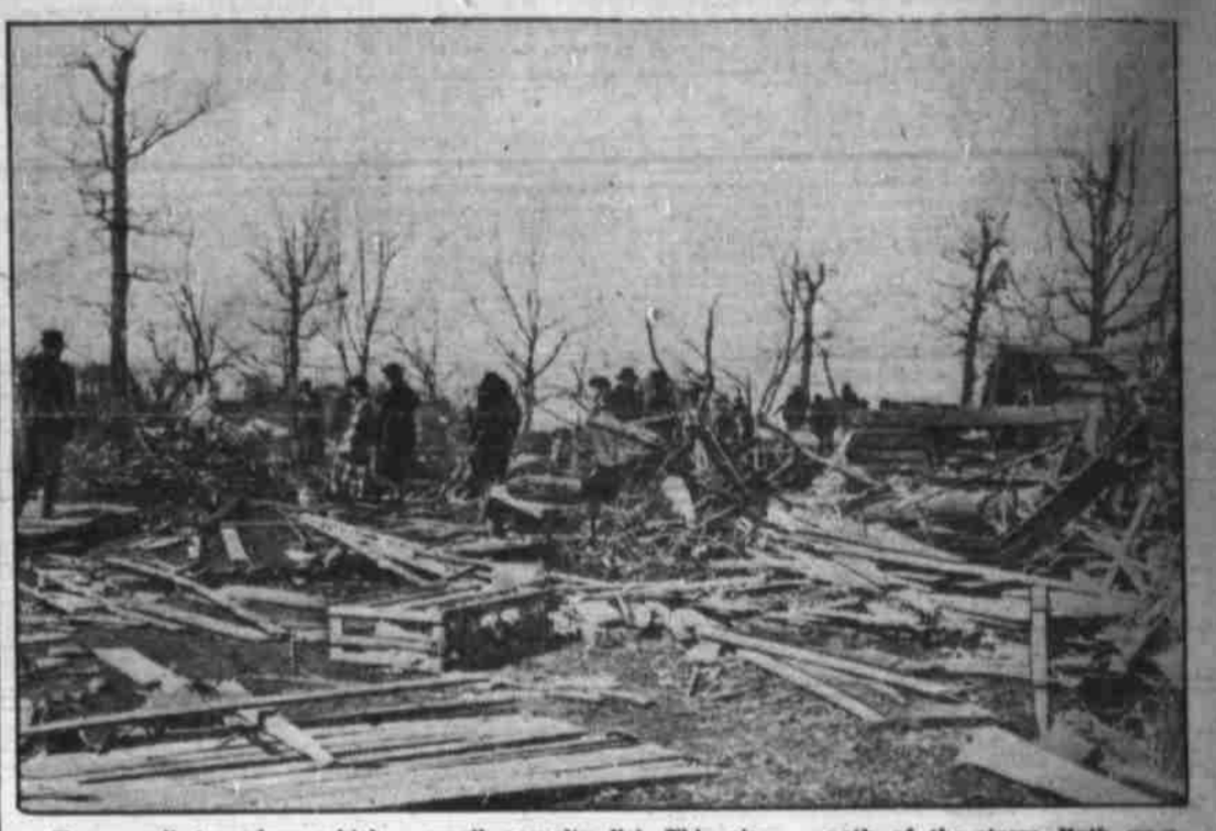
Two small tornadoes which swept through several south-west Missouri counties left heavy property damage, but a small casualty list. This view shows the leveled farm home of Mr. and Mrs. Charles Plank, near Rogersville, Mo., in the path of the storm. Both were injured seriously. (Associated Press Photo).
