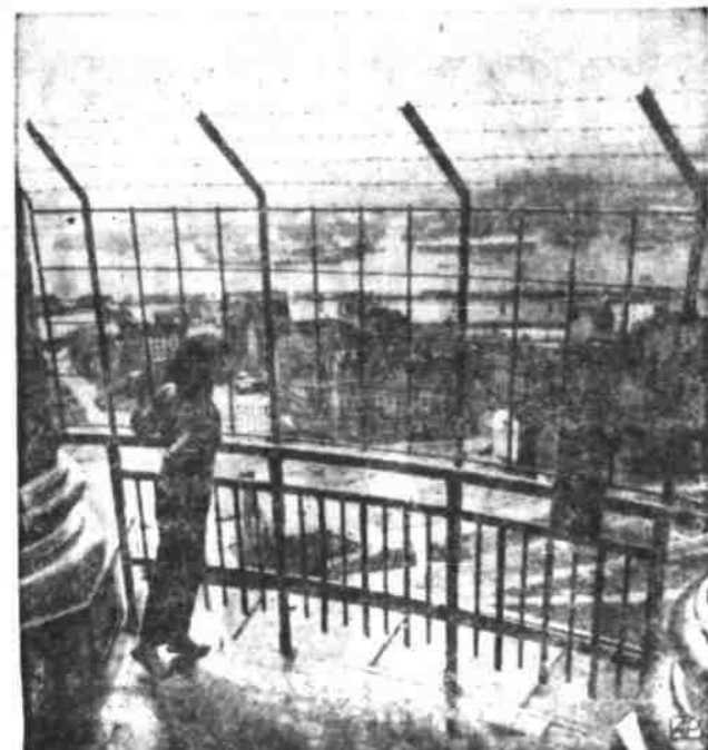
FENCING WITH SUICIDE — Addition to fence enclosing walk atop Hamburg's famous church spire, "Michel," is designed to prevent suicides from jumping from 433-foot tower.
