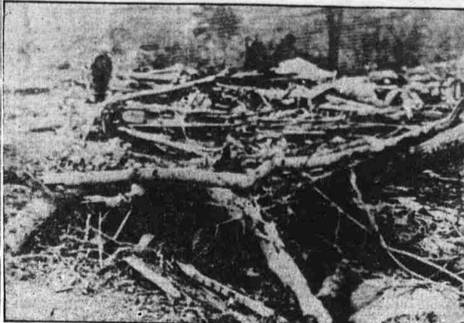
This Associated Press telephoto shows the wreckage of a house in Cartersville, Ga., in which seven persons narrowly escaped death. This was typical of destruction caused by tornadoes in several southern states.
