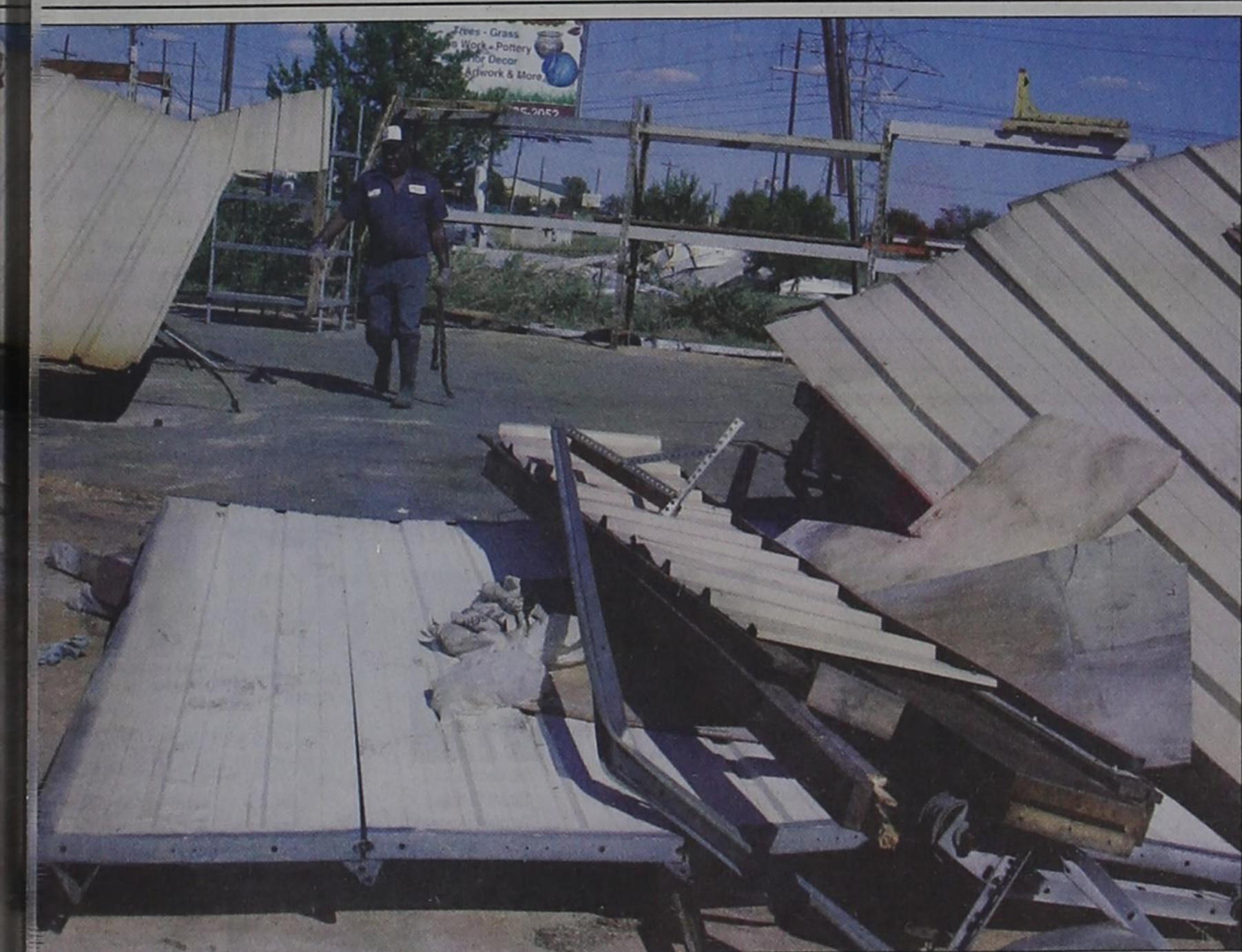
Rusty Jones assesses and cleans up the damage of Jayhawk Industrial Services on Friday, from the storm that rolled through the area on Thursday, October 2. The business is located at the intersection of Highway 276 and Gumbo Drive in Rockwall. Photo by Tim Burnett/Rockwall County News
