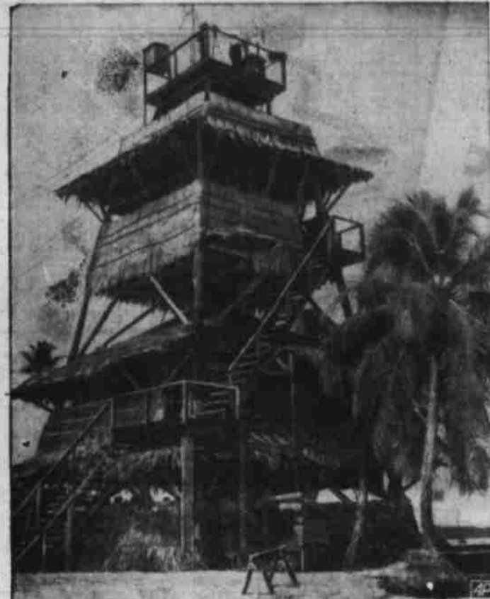
PAGODA TOWER —Despite its resemblance to a pagoda, this is really a flight control tower for a Navy FBY unit somewhere in the South Pacific. Built in three tiers, it has an observation platform at the top.
