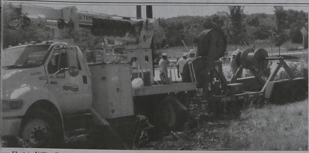
Electric Utility Construction survey the damage to their work truck after a fire. Crews were replacing electric cables along SH205 south of I-30 on Tuesday, July 29, when the truck, pulling a trailer with spools of cable, caught fire in the field and ignited the small fire. The workers used fire extinguishers until the fire department arrived to put out the fire and ensure the safety of the workers. Photo by Williams
