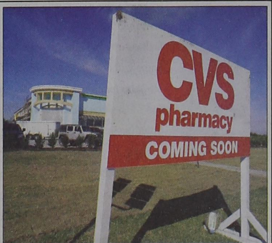
Located at the intersection of Lawrence Drive and Highway 740 in Heath, construction on the CVS Pharmacy is well underway. According to Heath Director of Community and Economic Development, Kim Dobbs, CVS is scheduled to open at the end of November.
