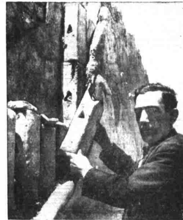
ANCIENT PLUMBING — Hollow tiles with vents which carried steam to heat walls of baths are among discoveries by archaeologists in new excavation at Pompeii, Italy.
