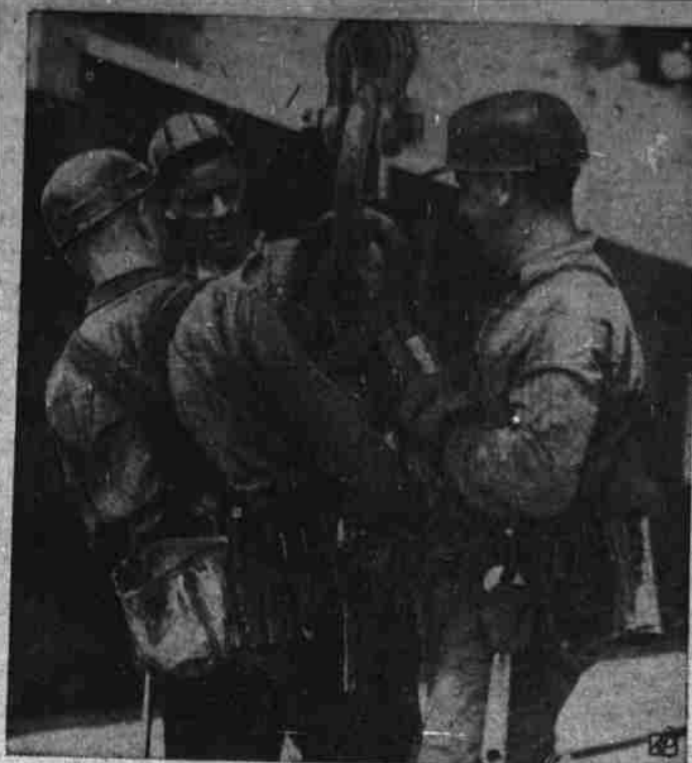
3 OF THE 3,235 workers who'll raise Grand Coulee dam to its full 550-foot height start to work along Columbia river.
