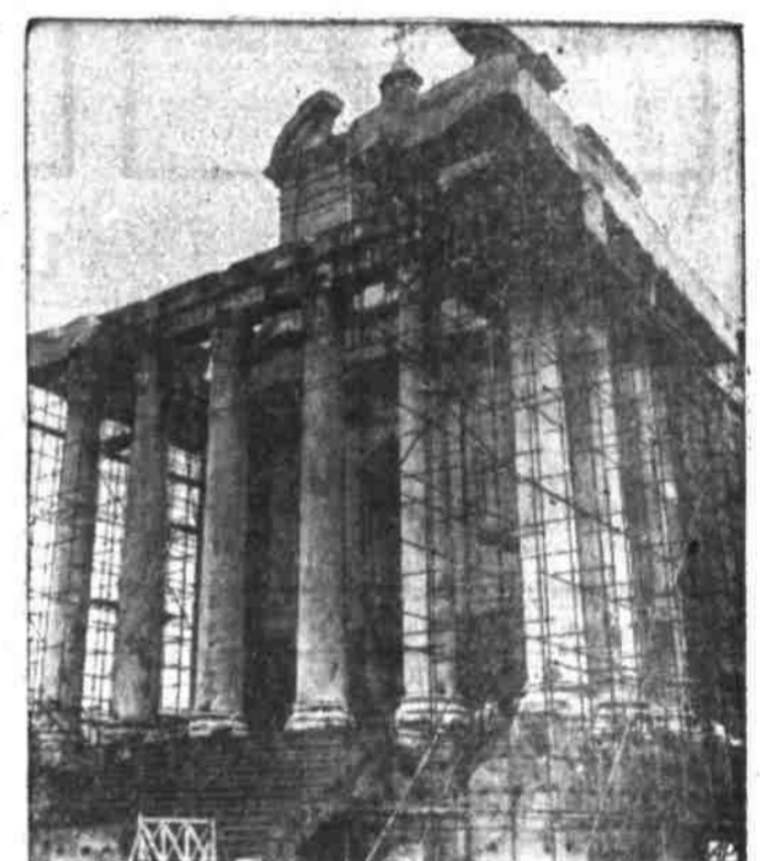
AN ANCIENT TEMPLE IS RESTORED — Portico and facade show restoration work in progress on the Temple of Antoninus and Faustina built in 141 A.D., in Rome.
