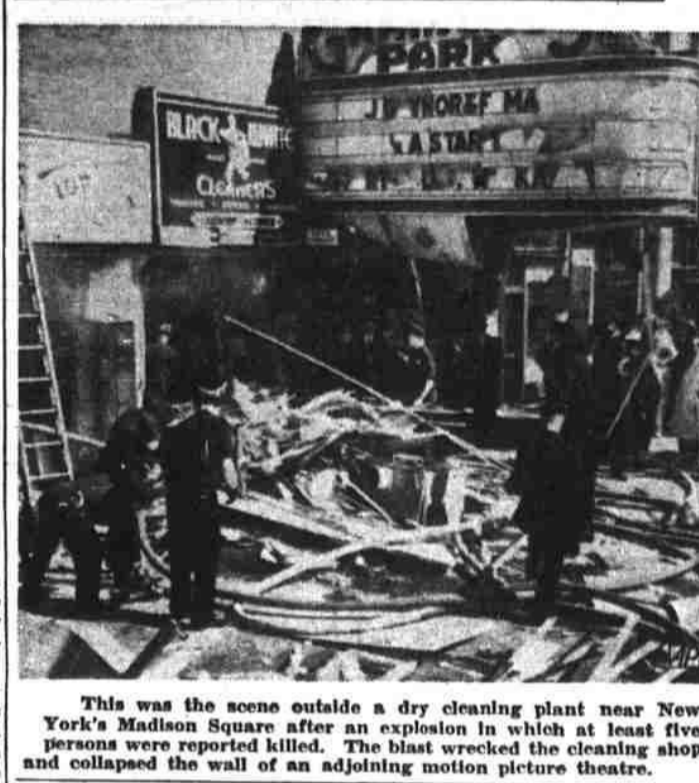
This was the scene outside a dry cleaning plant near New York's Madison Square after an explosion in which at least five persons were reported killed. The blast wrecked the cleaning shop and collapsed the wall of an adjoining motion picture theatre.
