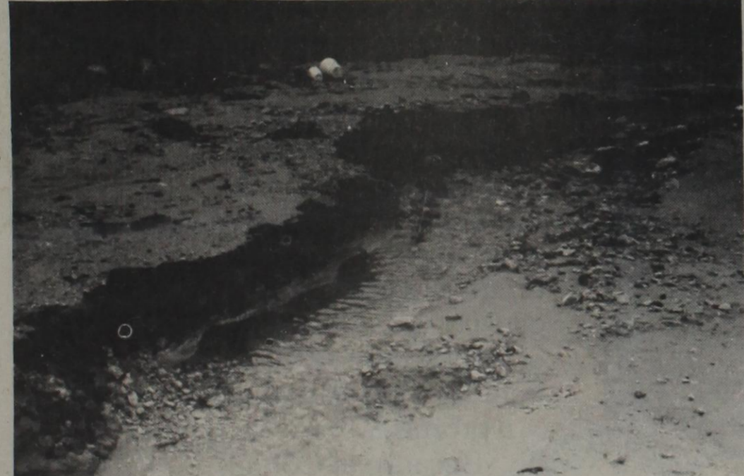
A common sight over a wide area after the flooding April 25-26 was damage the heavy rains caused to dirt roads. This is the east city limit of Rising Star north of Highway 36. City crews made emergency repairs the next day only to have their work undone when four inches of rain fell April 29-30.
