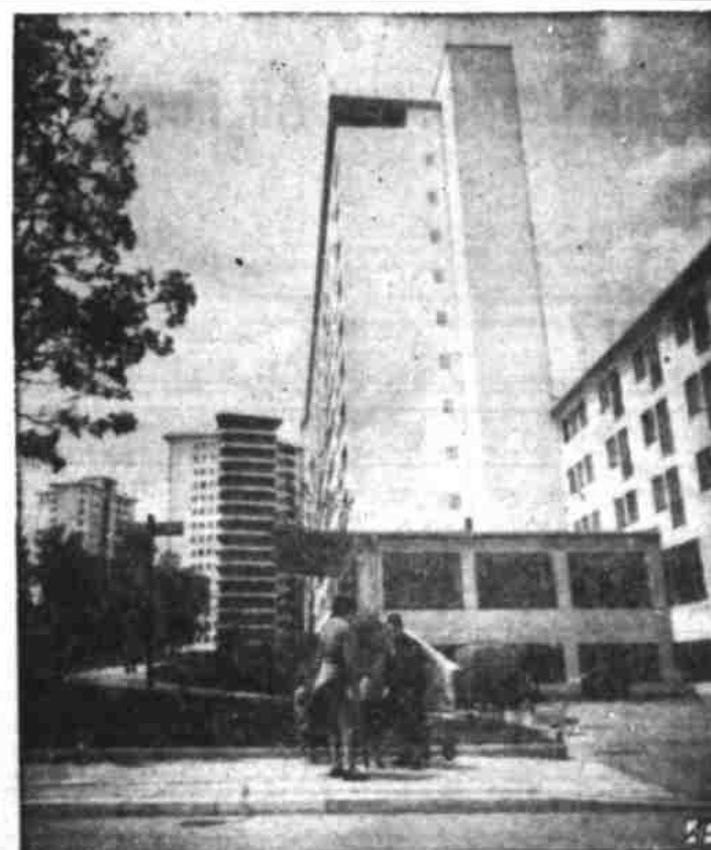
PROGRESS IN MUNICH — This 17-story office building tops blocks of apartments in modern district of Sendling, Munich, Germany, suburb. Project contains 569 apartments.
