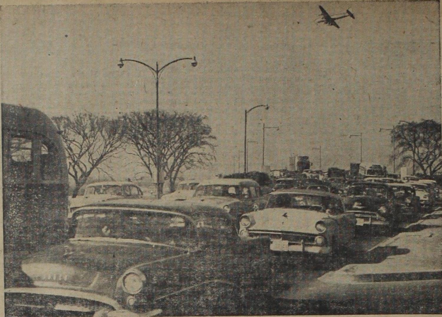
CIVIL DEFENSE EVACUATION would look like this with carefully controlled traffic moving one-way outbound from a threatened target city at a rate of up to 1,200 autos per hour per lane, except that cars would be carrying more people. All access to major surface streets would be controlled, traffic on cross streets banned. Reports indicate that some 32 million persons could be evacuated from 185 target areas in 1 1/2 hours by using this system. (Cameramen, Inc., Photo by Berkeley Payne)
