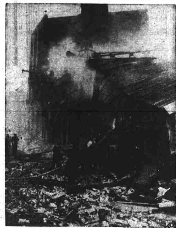
CHEMICAL PLANT BUILDING BLASTED APART—Two buildings at the Penna Industrial Chemical Corporation's plant at Clariton, Pa., were blasted apart Wednesday by a thunderous explosion of resin and oils.
