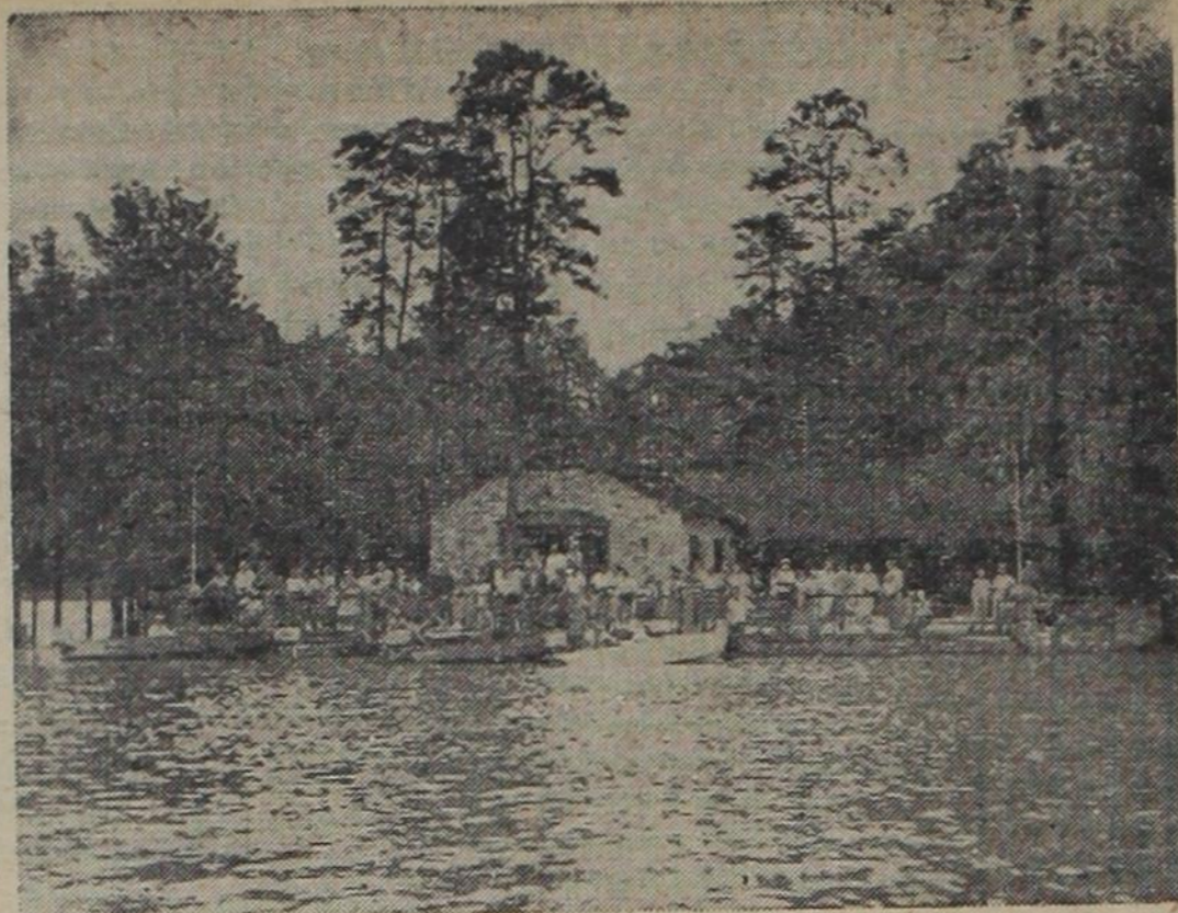
HUNTSVILLE STATE PARK is on a paved park road that leaves U. S. Highway 75 six miles south of Huntsville. The park now has a 300-acre lake behind a dam that was rebuilt last year. The spillway of the original dam was washed out by a heavy flood in 1940. Its replacement was financed by selling timber selectively cut in the park's 2,000-acre forest. During the idle period the lake was expertly managed to get the best fishing. It was opened to fishermen June 1, 1957. Photo by Frank Dobbs, Huntsville
