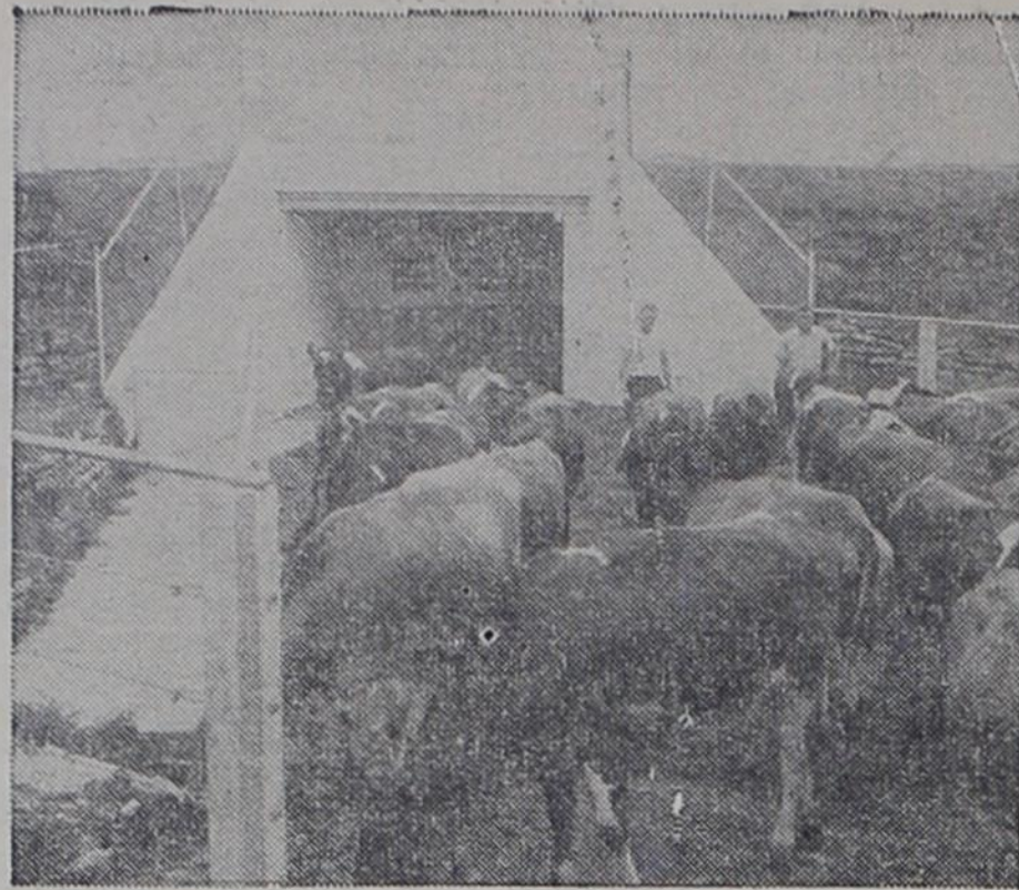
DAIRY COWS graze contentedly outside the entrance to an underground livestock shelter near Elkhorn, Neb., which was built by J. Gordon Roberts, president of Roberts Dairy of Omaha, to protect 200 Guernsey cows and three bulls from a nuclear attack. His dairy farm is only about 25 miles from Strategic Air Command headquarters near Omaha. In peacetime, the $35,000 shelter is used as a "loafing shed" for the cows to get out of the sun. Roberts, who has also built shelters for his family and employees, says he built the livestock shelter because "the American dairy cow is one of the best in the world. It took 300 years to produce this type of animal. It makes sense to preserve it if we can."
