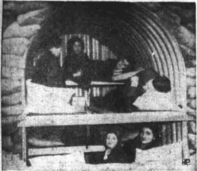
IT'S CRAMPED BUT SAFE—A London family shows how one of the small Anderson shelters can be used as a family dwelling during long air raid alarms. The British caption says the idea of equipping the shelters with bunks belongs to a London policeman. This shelter is capable of holding bunks for four adults and four children.
