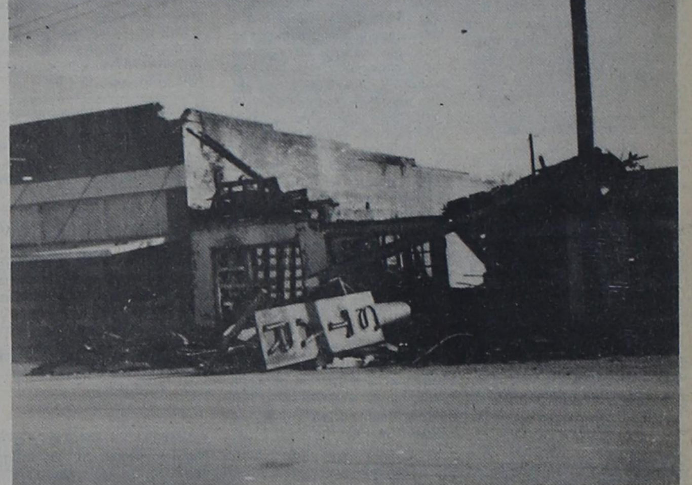
The old Star Theatre building was destroyed by fire on Saturday afternoon. (Photo by Edra Butler.)
