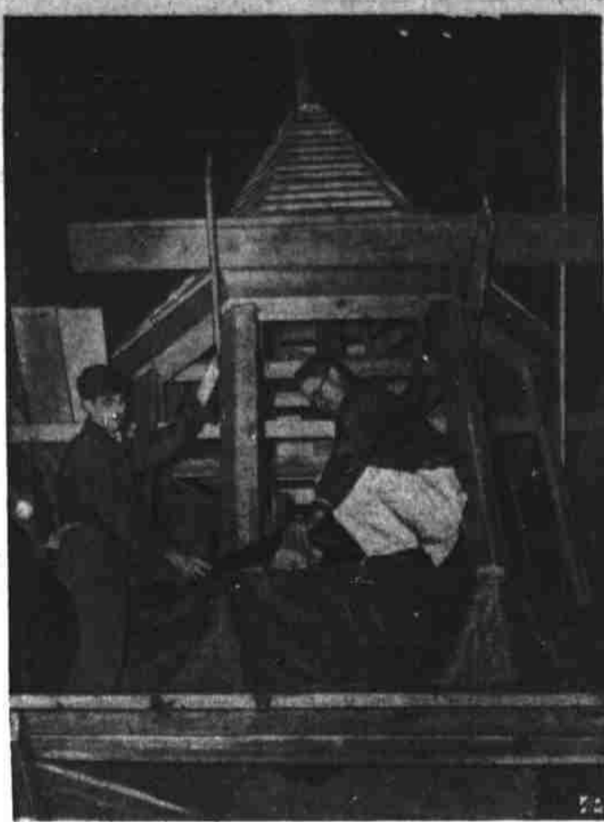
WILLING HANDS BUILD A CHURCH—As long as energy as they were short on cash, the congregation of the Missionhill Baptist church in Johnson county, Kansas, pitched in to build a 62x100 foot church topped by above belfry, on which the Rev. L. C. Pennington (right), pastor, and B. Cross labor. About 30 men, working week nights, built tiny $2,000 structure.
