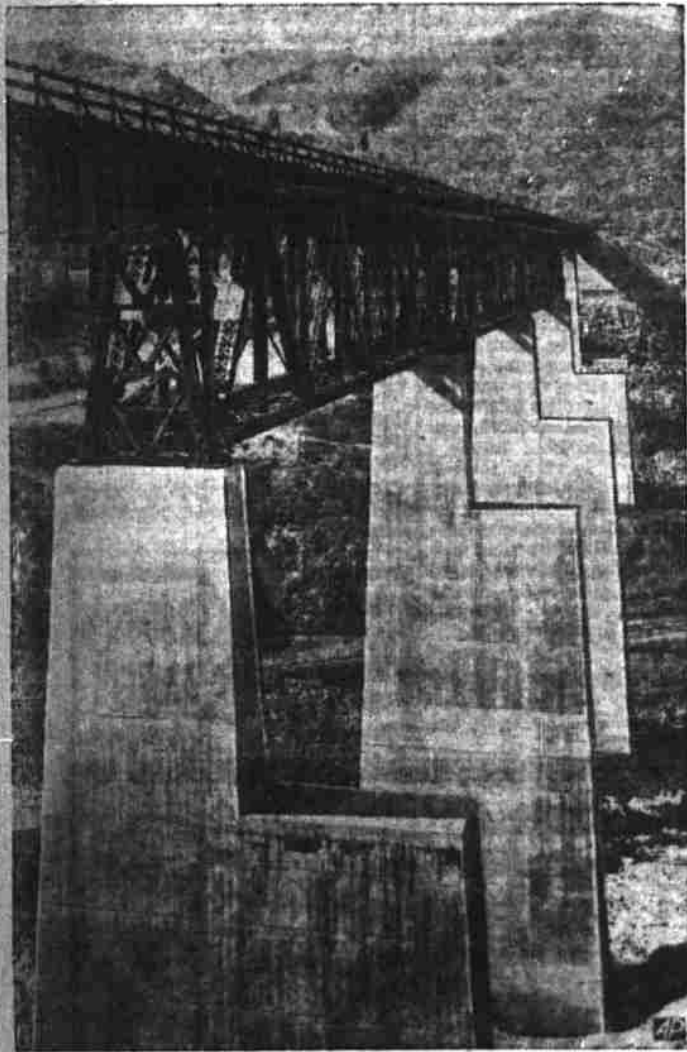
SHASTA UNDER WAY —Among the nine new bridges that will handle rail and motor traffic around Shasta reservoir in northern California is this, being built near Fullock. Shasta is part of the Central Valley river-control project. Another of the Shasta spans will be Pitt River bridge, 500 feet high; it will be the world's highest double-deck span.
