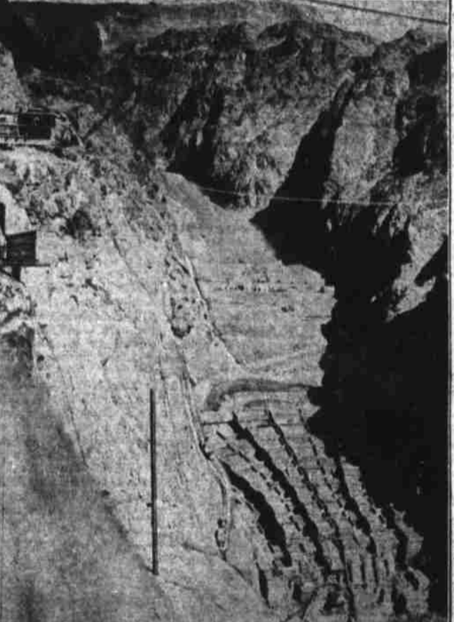
This comprehensive view of the foundation work on gigantic Boulder dam gives a hint of the vastness of the 1,000-foot gorge of Black canyon, where the Colorado river flows through southwestern Nevada, and into which thousands of tons of concrete are lowered daily by means of overhead tramways. (Associated Press Photo)
