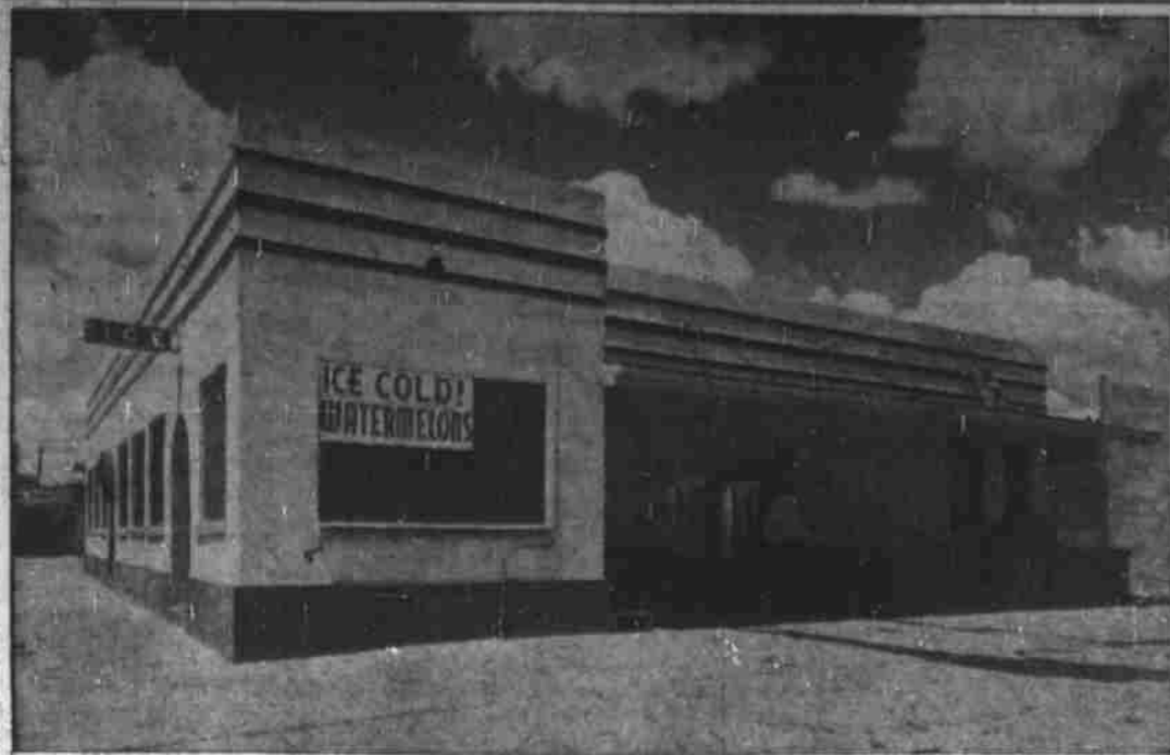
ICE DEPARTMENT of the new Banner Creamery plant is shown in the above photo. This dock, from which trucks are serviced, fronts on Young street, the east side of the new building. Banner has its own ice manufacturing department, and John Edgar is in charge of ice production.—(Photo by Kelsey).
