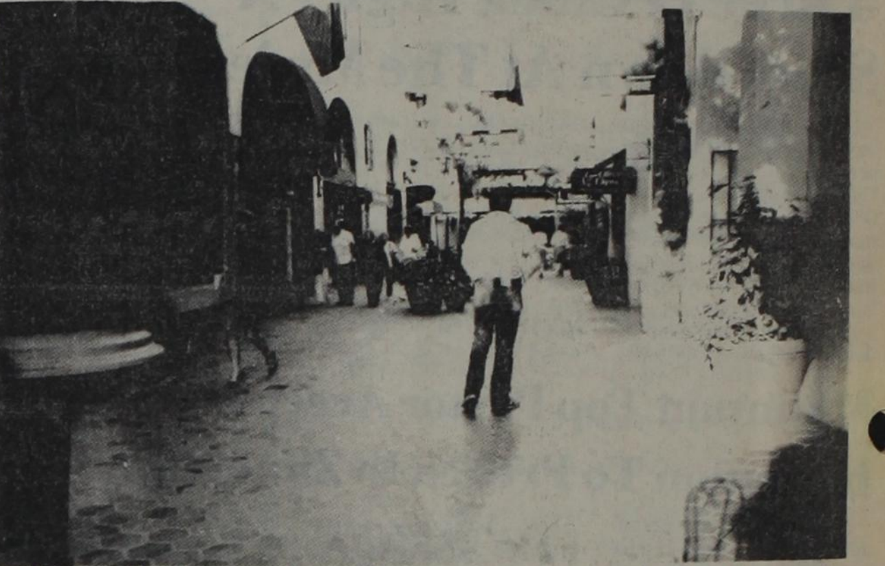
This mall in downtown Santa Barbara shows what can be done to beautify older buildings.
