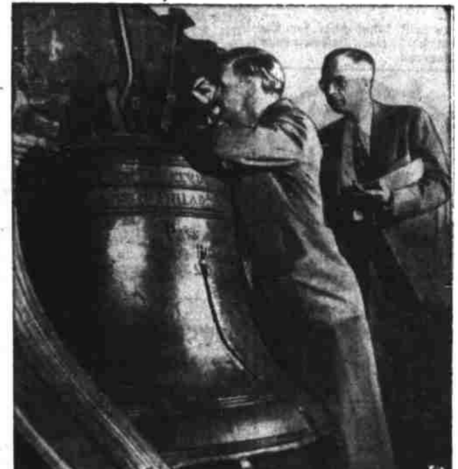
SUPPORT CHECK —Dr. B. Francis Kukachka, left, and Alan D. Fress, wood experts, check the century-old wood beam supporting the Liberty Bell in Philadelphia to determine if the beam can continue to hold up the 2,000-pound bell.
