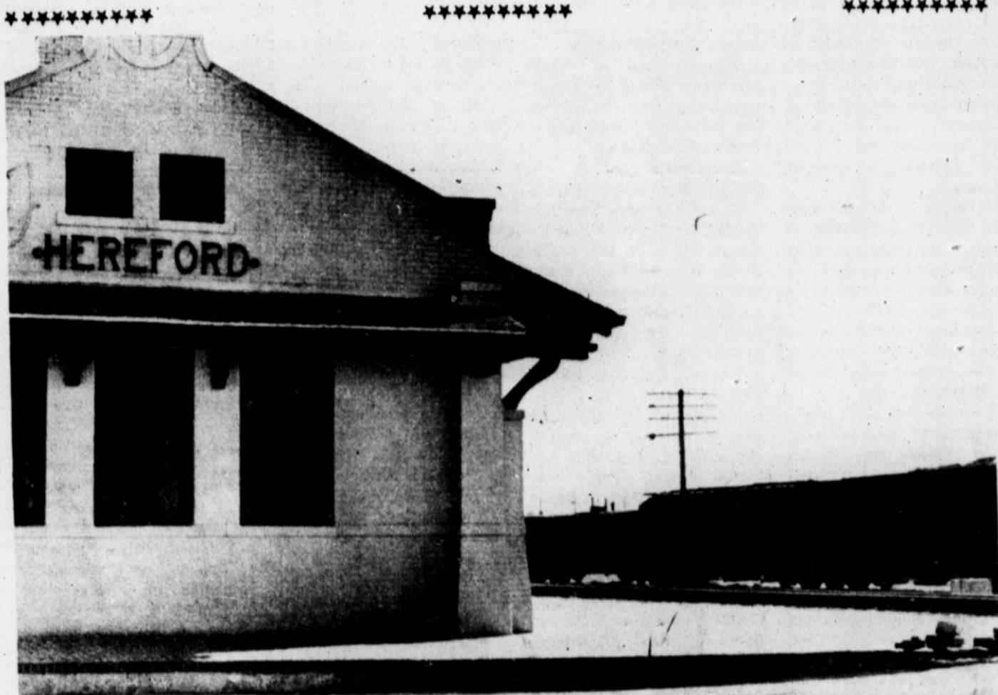
Vacant Train Depot
