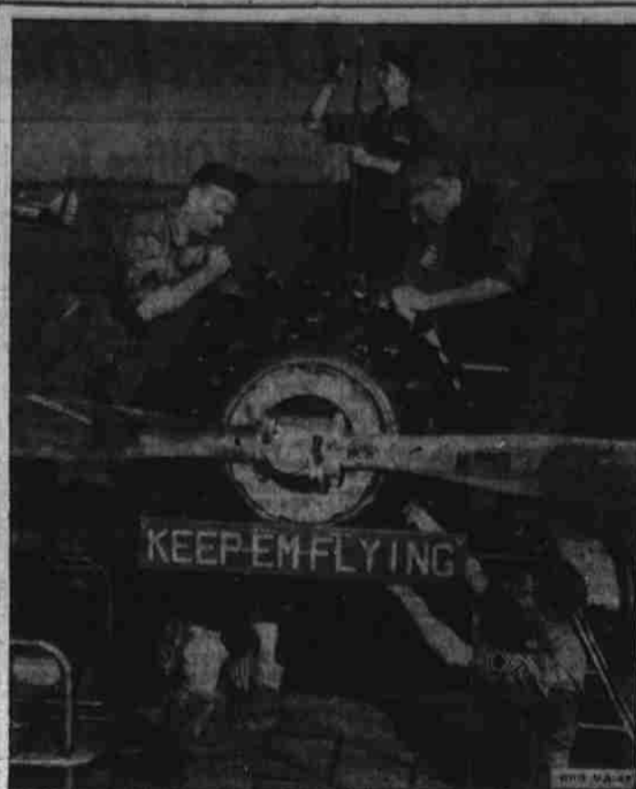
Ground crew members of the Army Air Forces now are literally hand-picked, for, under new Army plans, men with civilian experience as mechanics and radiomen are enlisted directly for the Air Forces and put right to work using the tools of their trade. The four mechanics above obey a "sign of the times" at Randolph Field, Texas, where they keep training planes in tiptop condition.
