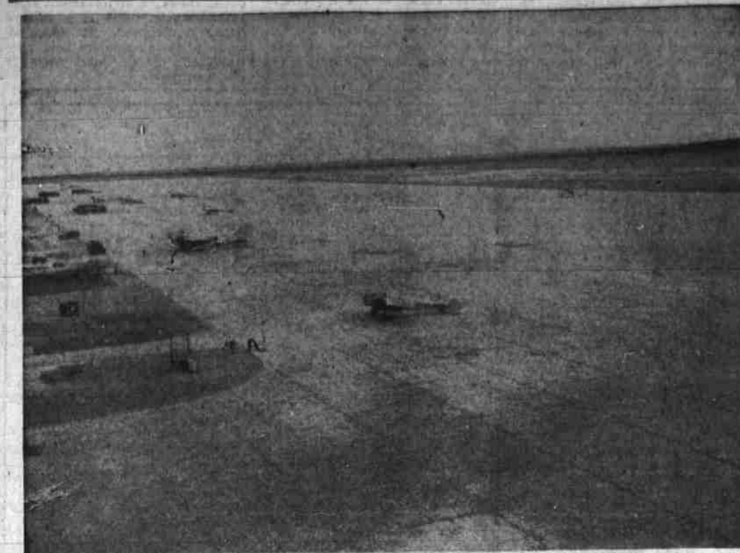
'Acres of Concrete' — Around two score acres of concrete went into the making of this gigantic apron for the Big Spring Army Air Forces Bombardier School. In addition to being a massive slab of heavy duty cement, the apron contains a series of imbedded iron rings to which planes may be lashed to the ground. So big is this facility that it requires special drainage outlets to care for since there would be no absorption from showers on its area.
