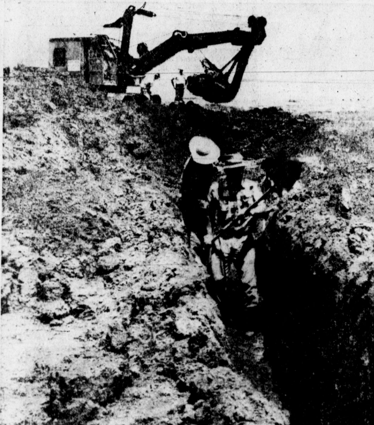
WATER STARTED DRAINING from the natural lake four miles north of Hereford Monday afternoon as Texas Highway Department workers tried to get rid of the four feet of water covering U. S. Highway 385. Ditches will carry the water to the vicinity of the city dumpground and then on to Tierra Blanca Creek. A huge backhoe dug out the channel leading into the lake. It is expected to take a week to drain the lake enough to allow through traffic. (Staff Photo)
