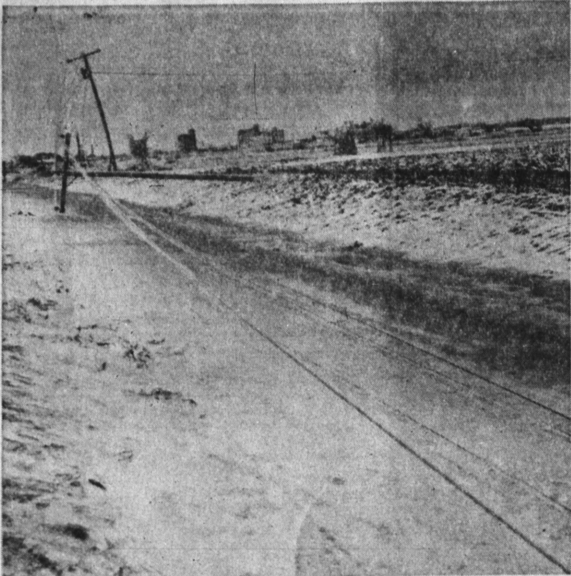
ICE-HEAVY power lines pulled poles to the ground this week to cut off much electricity leading to rural areas around Hereford. Repair of the lines continued as Wednesday brought thawing temperatures. (Staff Photo)
