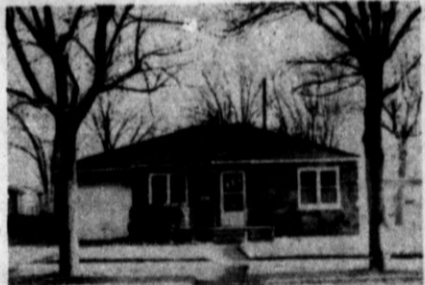
Just razoned for commercial business! Owner terms are possible on this stone house & large lot. If you need great exposure on 385 call Louie LeGrand. 4028
